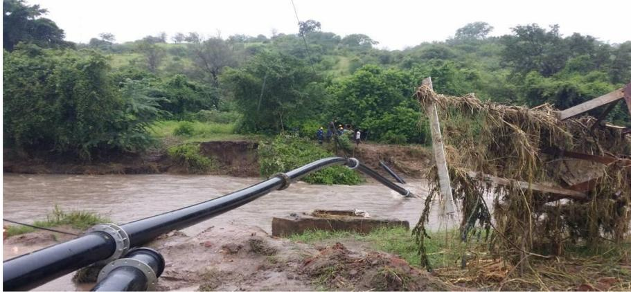
MCL staff and Management are collaborating and working with officials from SWASCO and the local officials to restore water to SWASCO's water treatment plant from Lake Kariba. The process to fully install the High-Density Polyethylene pipes is expected to be completed by Saturday evening. MCL is also assisting SWASCO in transporting pipes from outside the district to Maamba to replace washed away sewage pipes.
